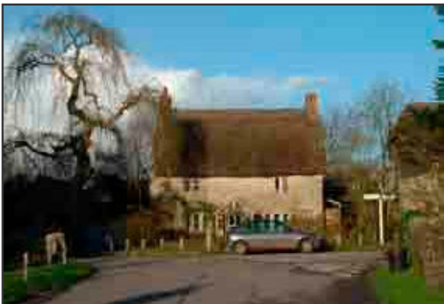
Limestone and thatch are typical of the villages, for example at Teffont Magna.
